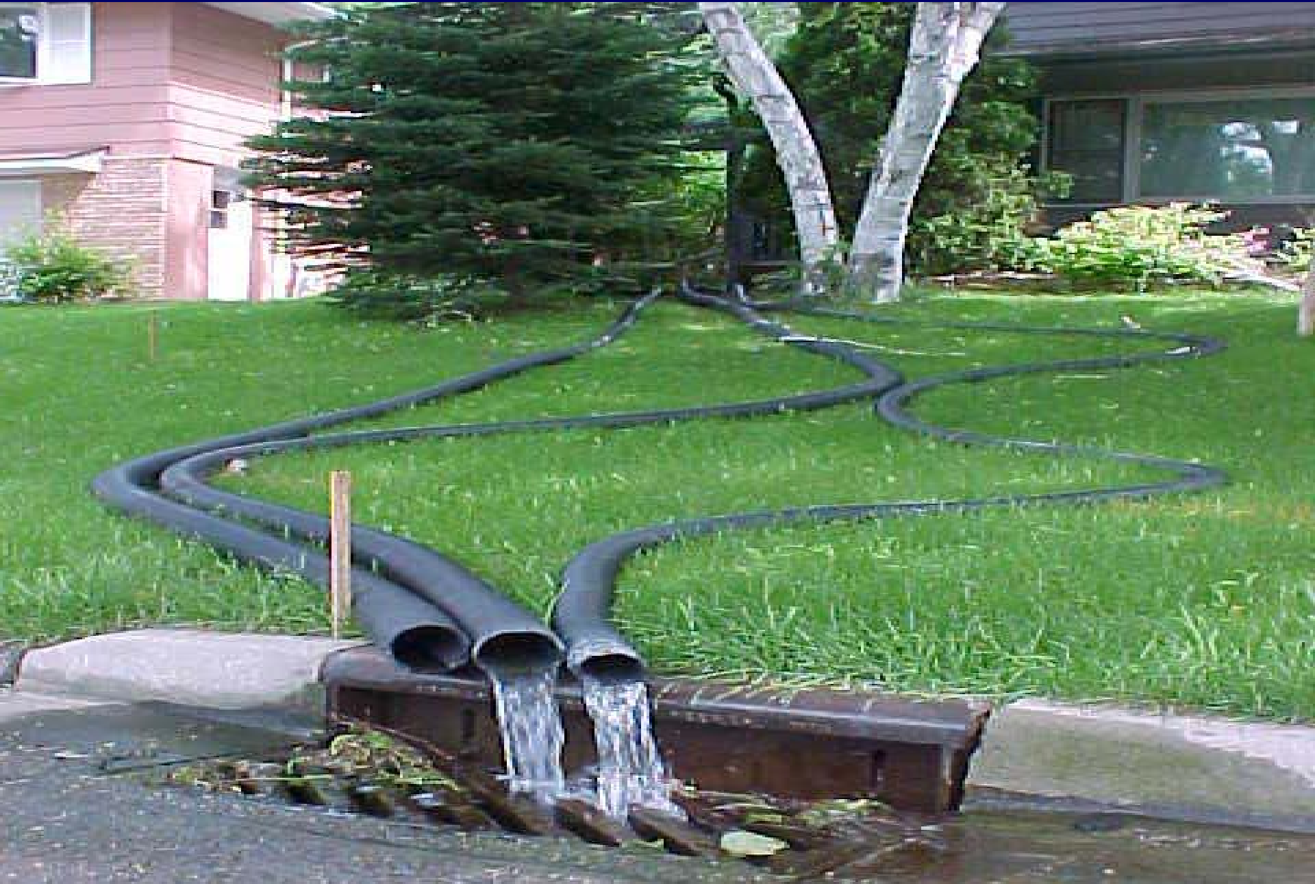
Water Being Pumped To The Storm Sewer From The Basement Of A Home Located On The Decorah Edge
