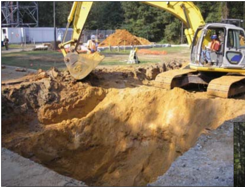
TCE Source Removal adjacent to Radar Tower
