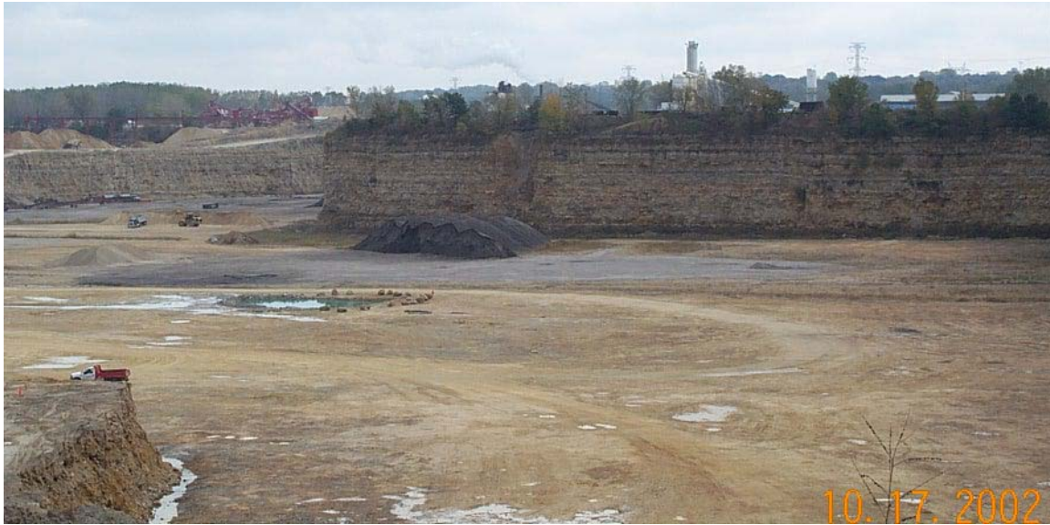
Figure 2.2. Kraemer quarry site photograph.
