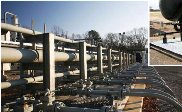
Well production manifold to allow individual testing of wells
