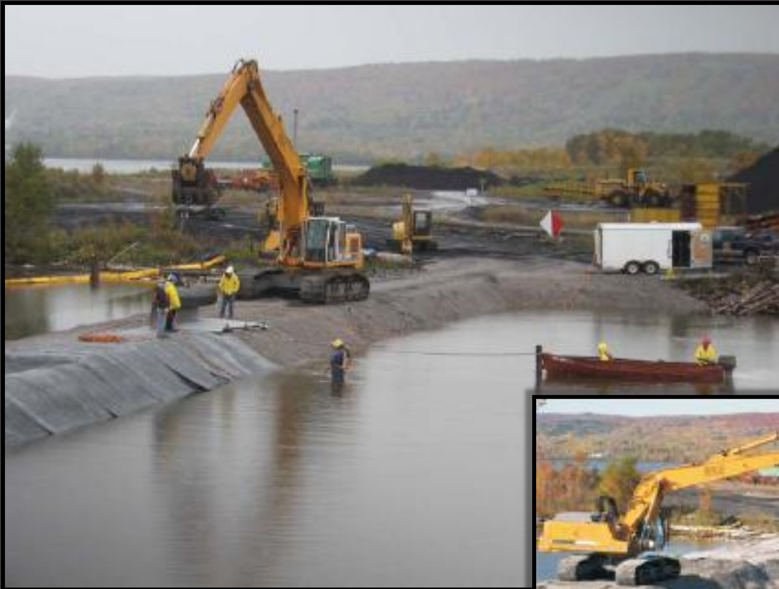
Clay Mat & Ballast Installation
