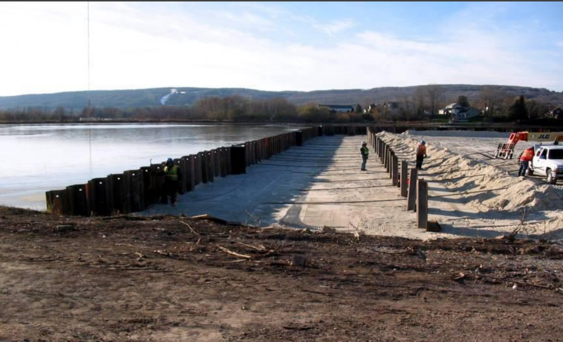
Installing Sheet Pile Wall Tie-backs
