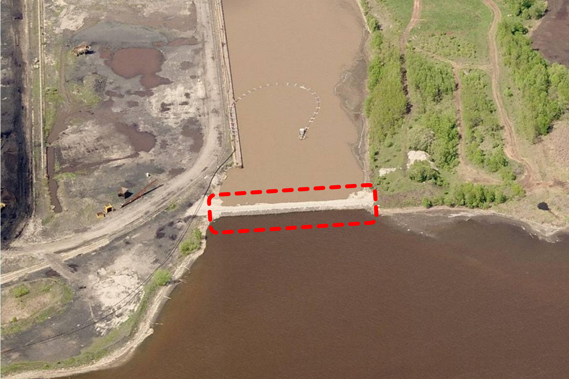
Cad End Dike Removal
