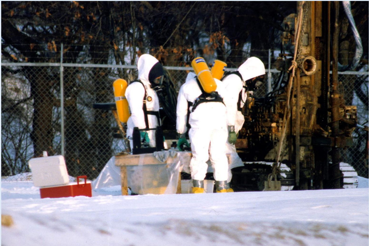
Drilling operations to verify the status of the Bruin Lagoon hazardous waste cleanup.
