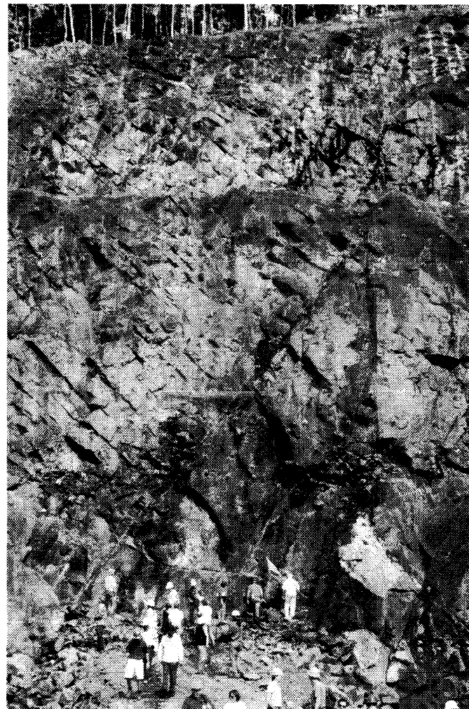
—Rock Bolts at Silver Cliff Tunnel
