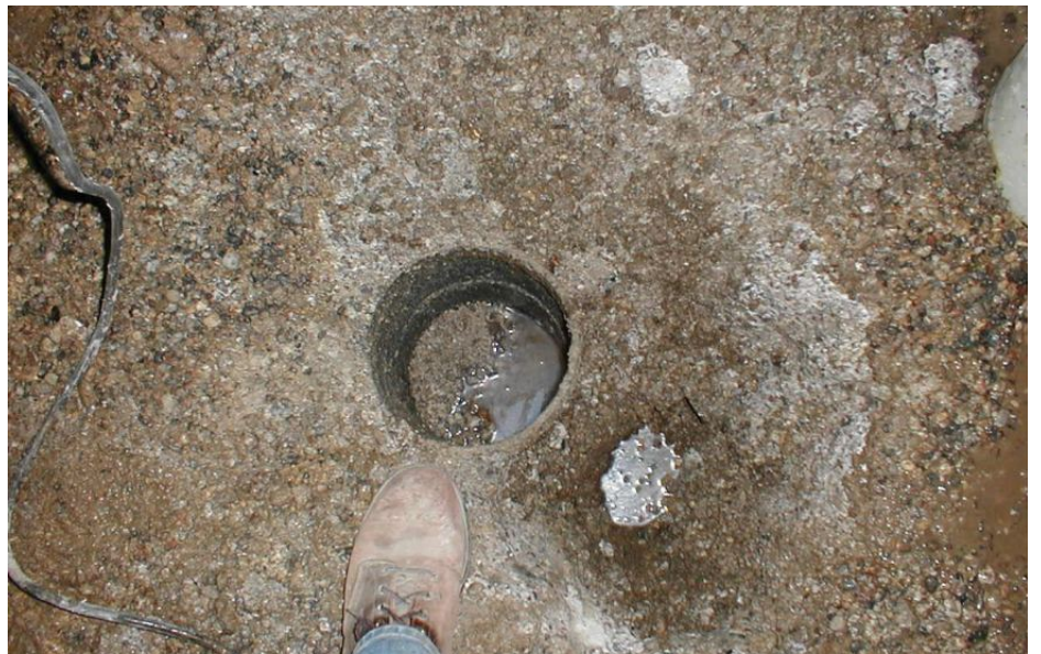
Abandoned 8-inch diameter railroad well improperly sealed with gravel and cement
