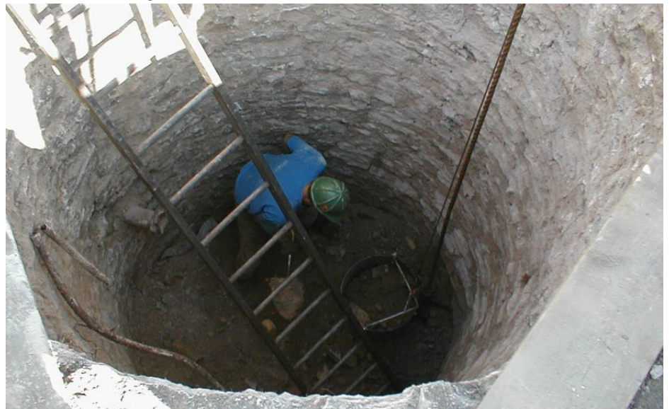
Well contractor, John Johnson, removing demolition debris from well pit
