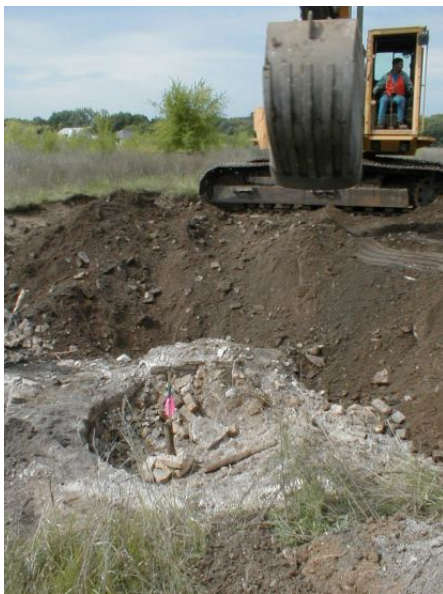
Eight foot diameter well pit found during excavation
