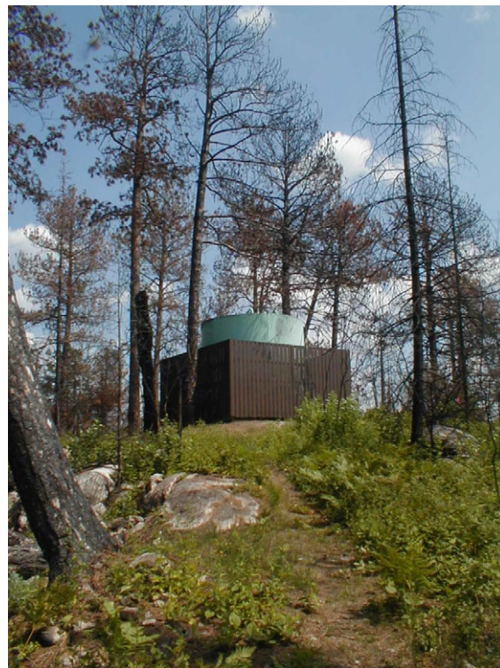
Figure 2: The steel storage tank was almost unscathed.
