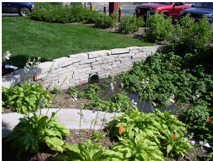
Example of a rain garden on the St. Paul campus of the University of Minnesota
