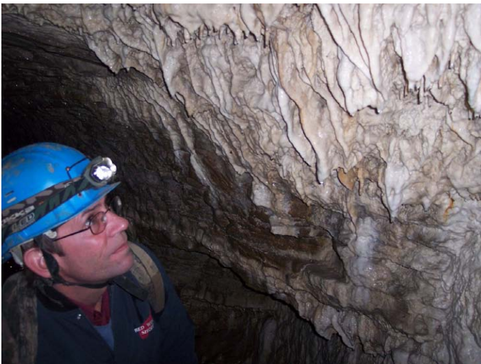
Figure 1. Flowstone deposits in the Bluff Street tunnel.
