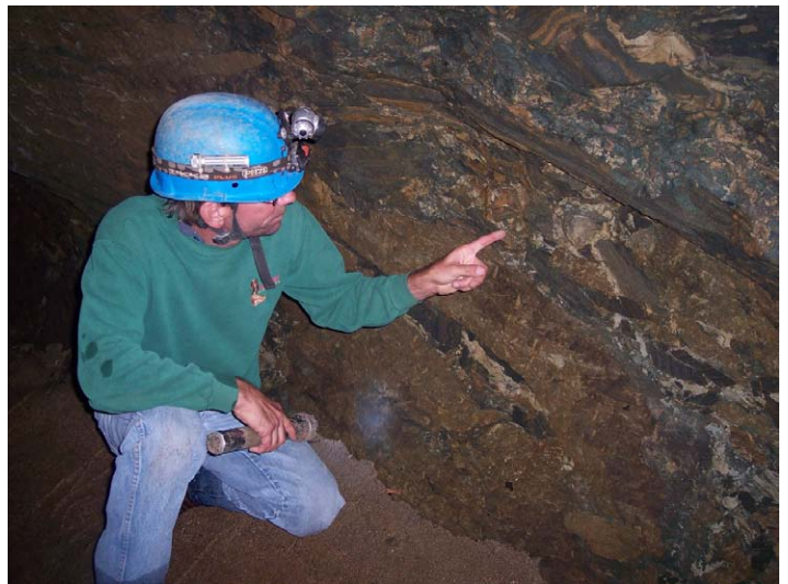
Figure 2. Red Wing fault breccia in the Bluff Street tunnel.
