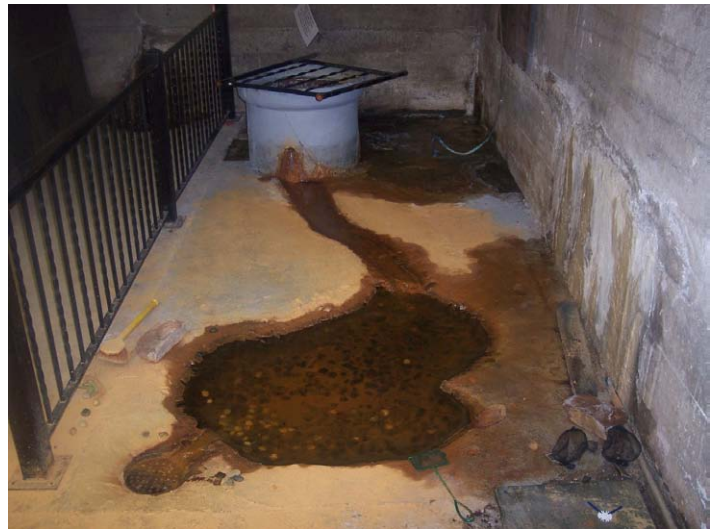
Figure 4. Basement floor drain, a supposed window into the Jordan River.
