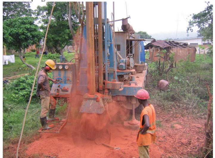
Drilling a well in a rural community in Ghana.
