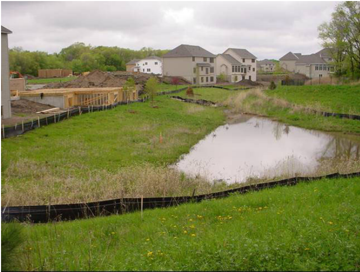
Figure 6. Despite over 30 feet of underlying granular soils, turf placed on top of this basin became the restrictive layer.
