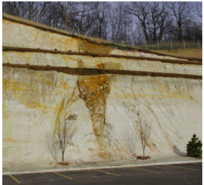
Possible paleo-karstic feature associated with fracturing in the St. Peter Sandstone, Rochester, Minnesota.
