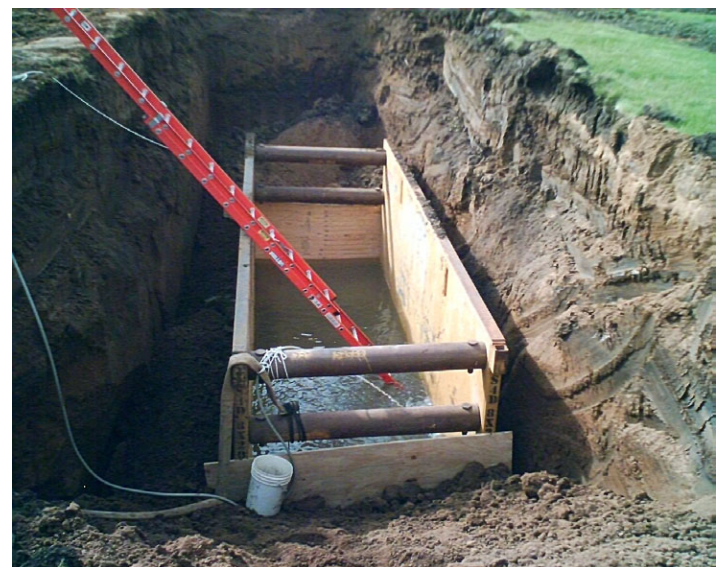
Figure 4. Infiltration pit test about 10' deep using a 6' x 20' trench box with plywood completing the sides.
