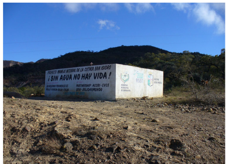
— A water supply tank in the San Isidro valley. 'Sin Agua No Hay Vida' means there is no life without water.
