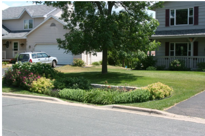
Figure 1: Bioretention cell in residential area. Note curb-cut where stormwater enters from street. (Photo: LeFevre)
