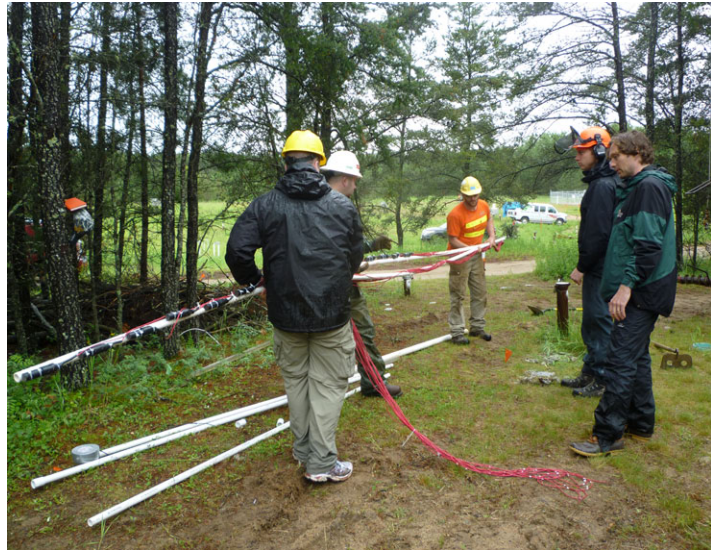
Deploying a geophysical array at the Bemidji site.
