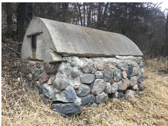
Fig 2. The stone springhouse on Skalbeck's Spring Farm. Photo by Greg Brick.
